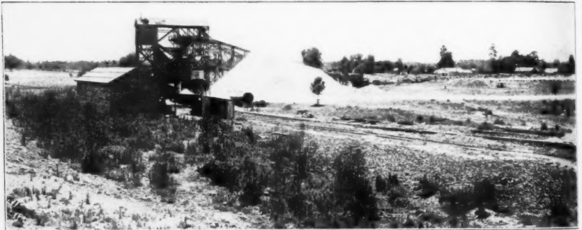
Crushed Stone Plant Number Two
